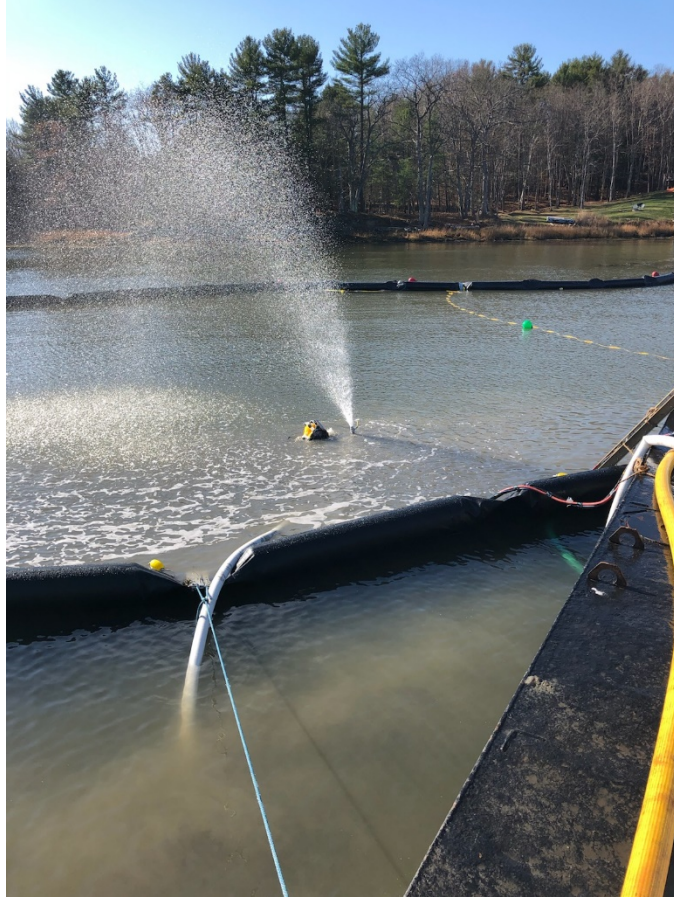
Diver burial in less than three feet of water within the turbidity barrier. Hand jet tool is “T” shaped with pressurized water out of both ends of the tool such that water shoots directly skyway (i.e., spouts) when held in certain positions at low water. Photograph taken by Durocher Marine from the diver barge located immediately adjacent to the turbidity curtain (11-15-19).
