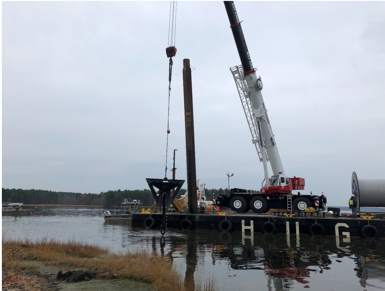
Anchor removal on eastern tidal flat (11-11-19).
